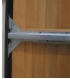
Strong steel lateral bracing with steel corner joints
